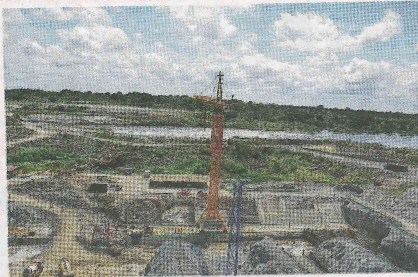
Karuma dam is 11 months to the completion deadline
